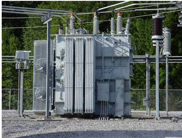
Figure 9.20: Substation transformer.
